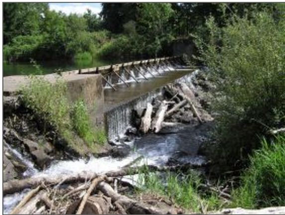
Brownsville Dam bedrock chute before removal
